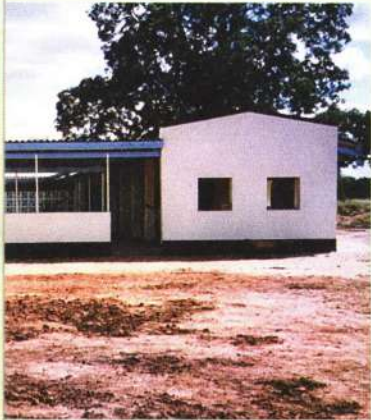
The newly built clinic.
