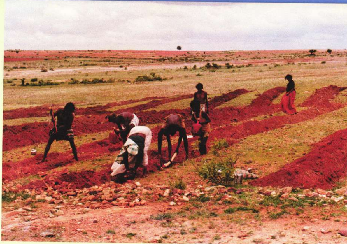
Trenches act as temporary drains to prevent runoff and erosion.
